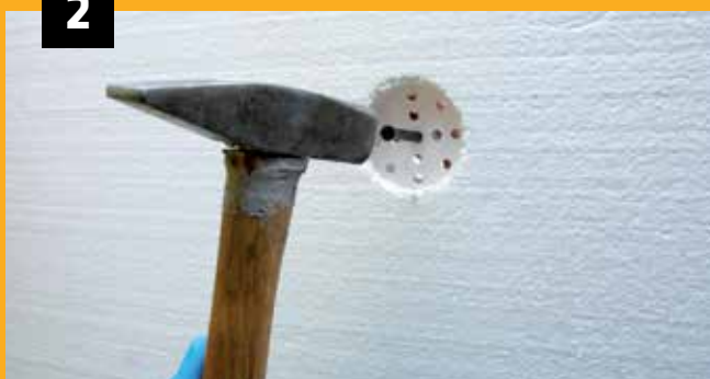
Dodatno pričvršćivanje EPS izolacione obloge Additional fixing of EPS insulation boards - anchoring
