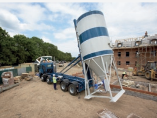
Dry-mortar silo at the job site with Sika powder additives
