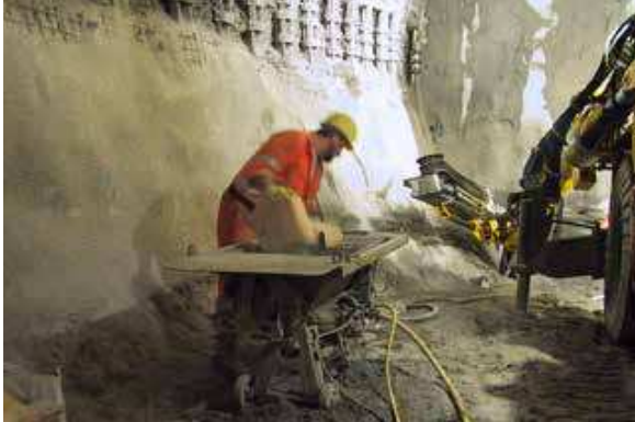
Temporary excavation stabilizing with dry sprayed mortar.
