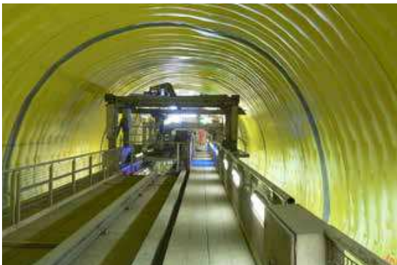
Durable waterproofing systems applied after stabilising with sprayed concrete and before the inner segment concrete lining.
