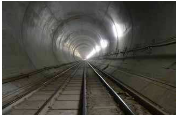
Inner segment concrete for durable final lining of the two main tubes.
