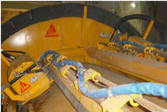
Sprayed concrete stabilisation behind the excavation with wet sprayed concrete in the TBM section.
